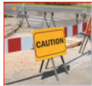
Figure 11 sign to show hazard areas
