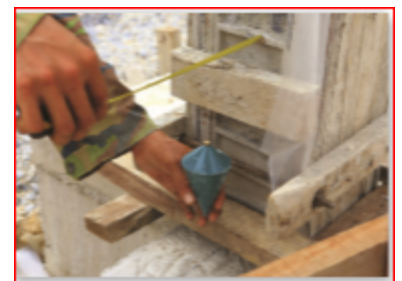
Figure 17 using plumb bob to check vertical alignment
