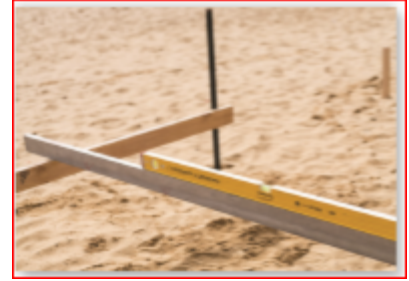
Figure 18 using straight edge to check horizontal line
